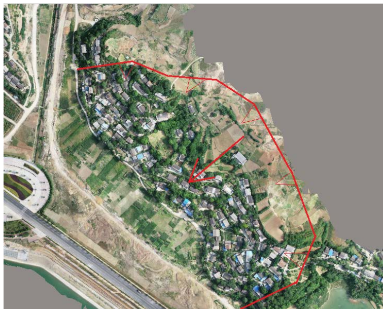
Figure 1. Panorama view of the landslide area 图 1. 滑坡区全景图
