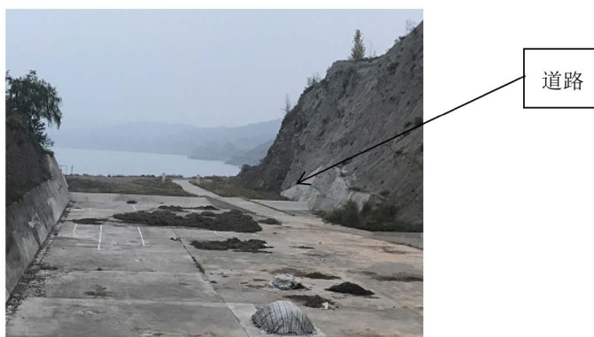
Figure 2. Road at the end of the spillway 图 2. 溢洪道末端交通道路
