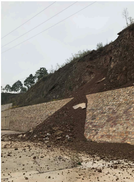
Figure 1. Side of spillway 图 1. 溢洪道边坡
