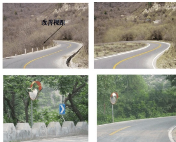
Figure 7. Improvement of visibility 图 7. 改善视距
