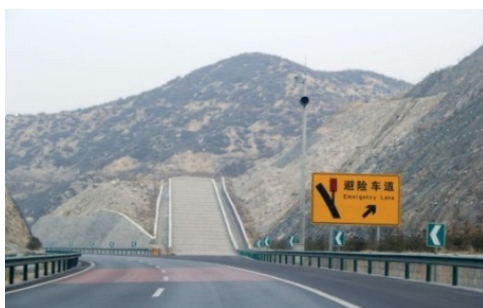
Figure 8. Truck escape road 图 8. 避险车道
