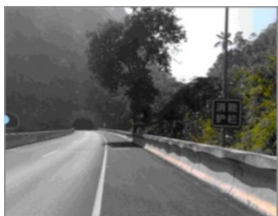
Figure 11. Energy dissipation and deceleration barrier 图 11. 消能减速护栏
