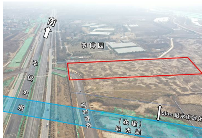
Figure 2. The present land use map for Yudou vehicle base 图 2. 鱼斗车辆基地场址现状图
