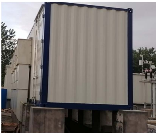
Figure 7. Installation drawing of the lower air inlet site 图 7. 下进风现场安装图
