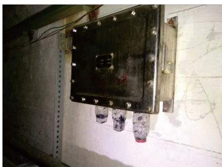
Figure 1. Grounding wire stolen picture
