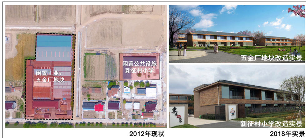
Figure 6. Comparison of idle industrial and public facilities before and after reconstruction 图 6. 闲置工业和公共设施地块改造前后对比图
