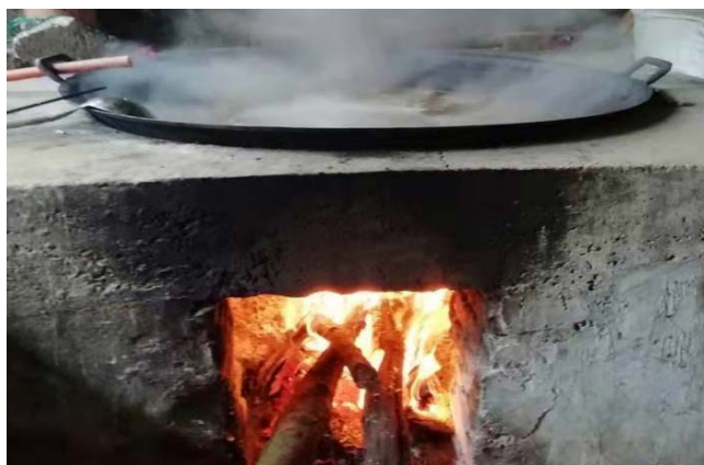
Figure 4. An earthen stove for burning firewood in rural houses 图 4. 农村住宅中烧柴的土灶
