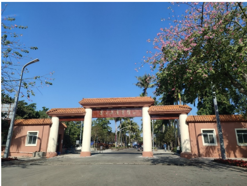
Figure 12. Real view of the main gate after landscape enhancement in Zhanjiang Seaside Hotel
