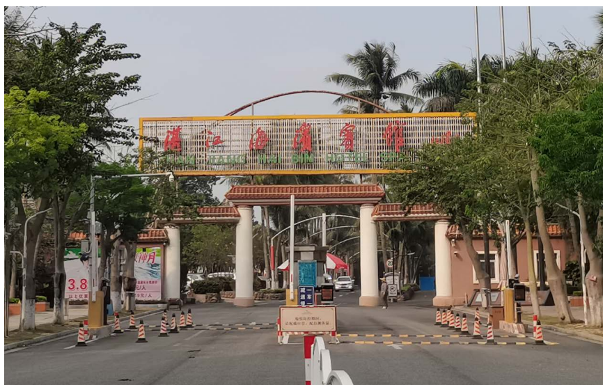
Figure 11. Real view of the main gate before landscape enhancement in Zhanjiang Seaside Hotel
