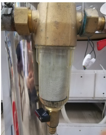
Figure 2. Cathode-back filter (internal corrosion cell) 图 2. 阴极后置过滤器(内置腐蚀电池)
