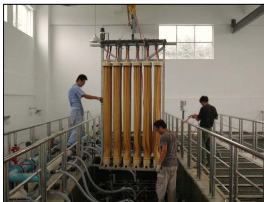
Figure 4. Installation of the hollow fiber membrane
