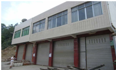
Photo 7. w2 windows and doors still can be freely opened, no large cracks, judged to be intact 照片 7. w2 门窗仍可以自由开启，无大的裂缝，判断为完好建筑
