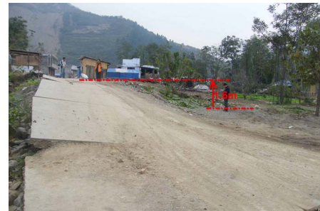
Photo 6. NB-6 thrust dextral, vertical dislocation 1.6 m, located at Hejiaba of Nanba town, Mirror to N40°E 照片 6. 南坝-6 逆冲右旋, 竖向位错 1.6 m, 位于南坝镇何家坝村, 镜向 N40°E
