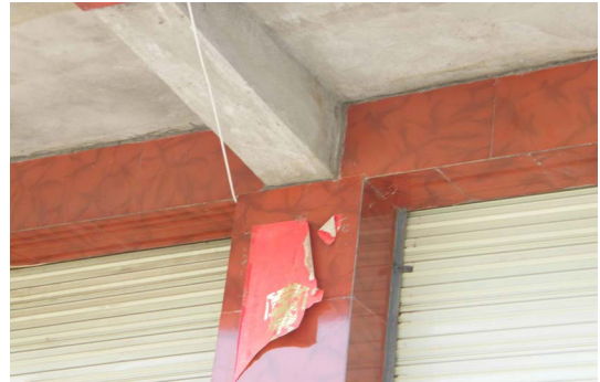
Photo 9. w6-1 the detail part of Photo W6, there is not cracks on beam and column 照片 9. w6-1 照片 w6 的细部图片，梁柱无裂纹
