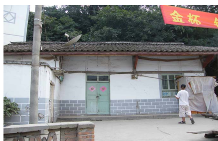
Photo 11. q9 window glass broken, tiles shrunken, but the whole structure largely intact, judged to be slight damaged building 照片 11. q9 窗玻璃碎裂，出现缩瓦现象，但结构整体基本完好，判定为轻微破坏
