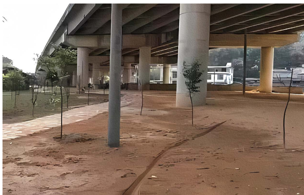
Figure 1. Liangmeng Village, Xinquan Town, Liancheng County plans to build a park square under the elevated bridge 图 1. 连城县新泉镇良盟村拟在高架桥下修建公园广场 ①
