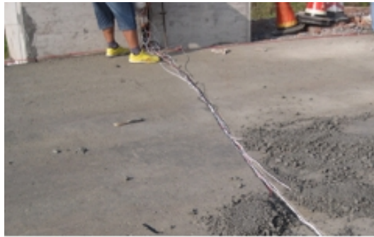
Figure 4. Embedding of road sensors 图 4. 路面传感器埋设
