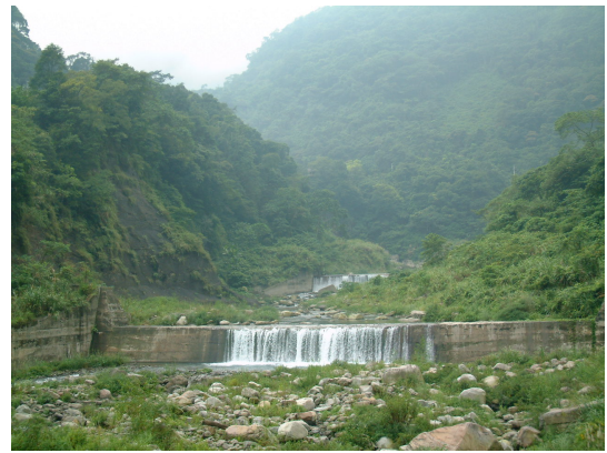
Figure 3. Sediment retention in enclosing section of East River 图 3. 东河护渔段拦砂坝
