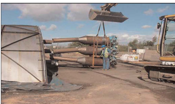
Figure 2. Fitting the burners [5]
