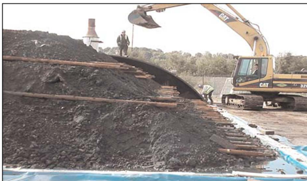
Figure 1. Moving the stainless steel panels into position [5]
