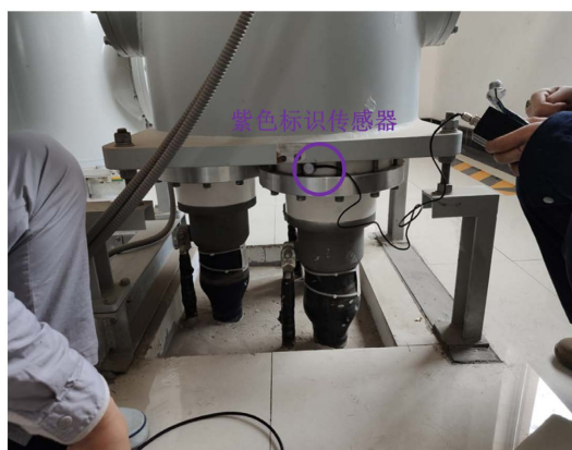
Figure 11. Field test photos of A phase cable terminal
