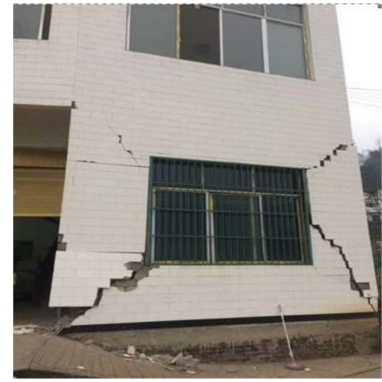
(c) 乐义乡黄金村砖混结构房屋墙体沿窗户 X 型开裂
