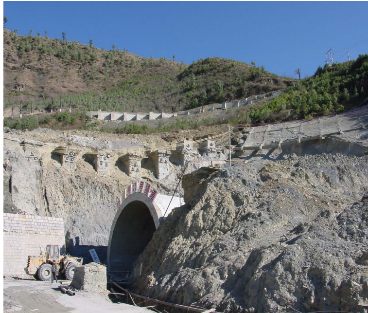
Figure 2. The exit of Baihejing tunnel 图 2. 白泥井隧道出口端
