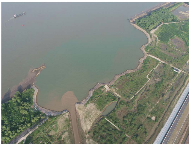
Figure 1. Aerial photo of the collapse of the bank in ZhiNan Village 图1. 指南村崩岸航拍照片
