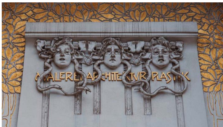
Figure 7. Exterior wall of the Vienna secession exhibition hall [8] 图 7. 维也纳分离派展览馆外部墙体[8]
