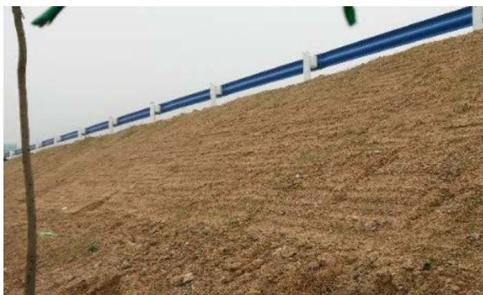
Figure 2. Construction site of vegetation-growing concrete 图 2. 植被砼施工现场
