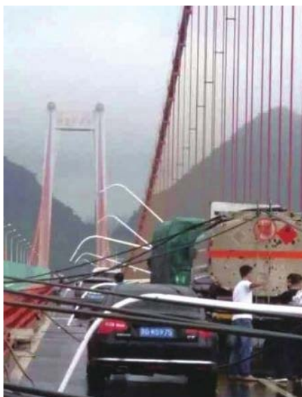
Figure 2. Gale disaster of Guanling Bridge 图 2. 关岭大桥大风灾害
