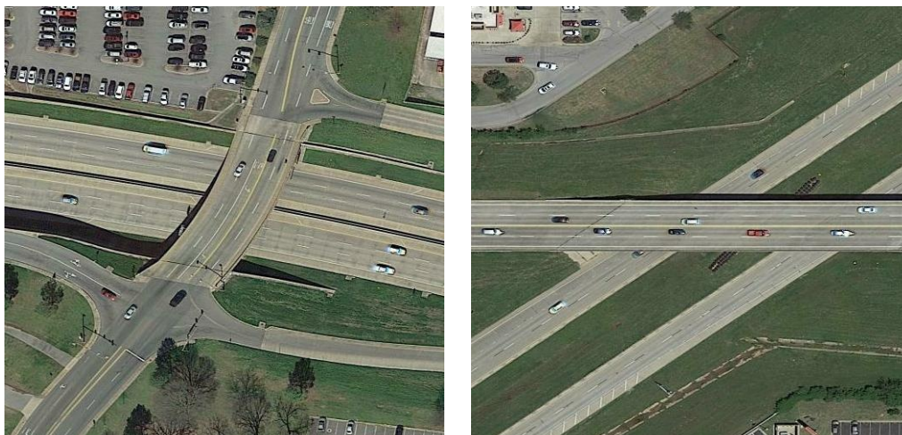
Figure 16. Bridge (left) and overpass (right) 图 16. 桥梁(左)与立交桥(右)
