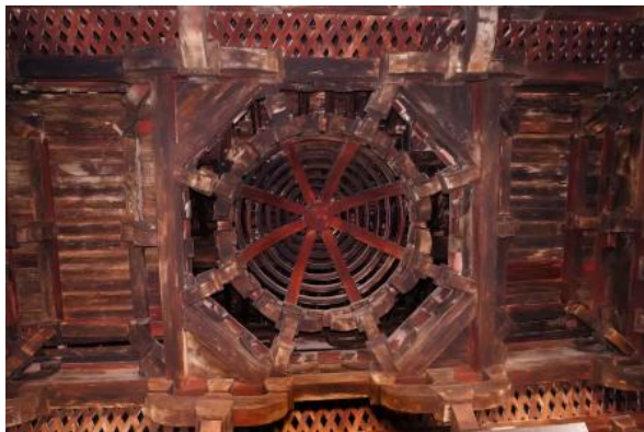
Figure 3. Bucket eight caisson: Baoguo Temple, Ningbo 图 3. 斗八藻井——宁波保国寺③
