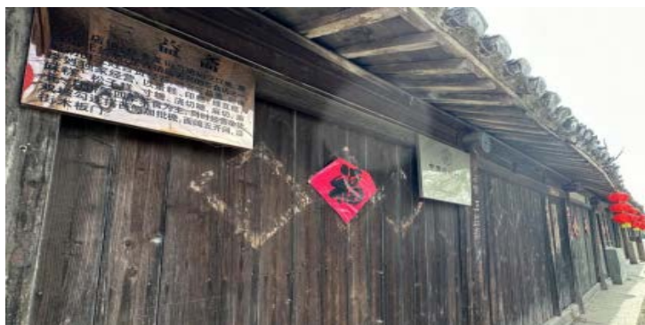
Figure 5. Low rise street style shops 图 5. 低层沿街式商铺
