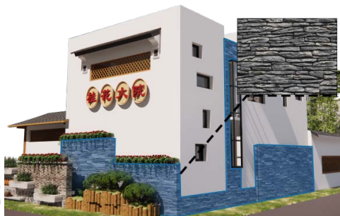
Figure 6. Schematic illustration of the exterior finish effect of shale 图 6. 页岩外饰面效果示意
