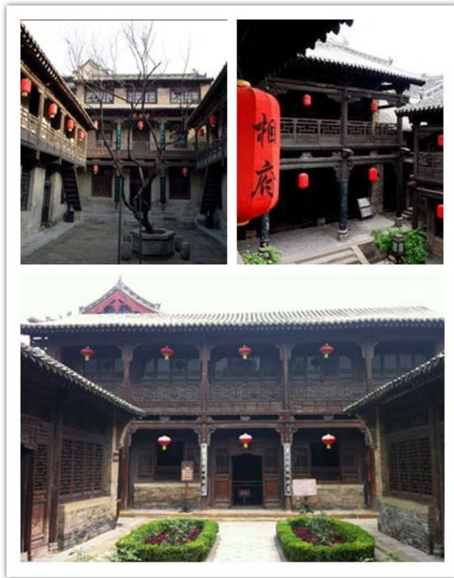
Figure 6. Southeast Shanxi storey courtyard characteristic chart 图 6. 晋东南楼院特征图
