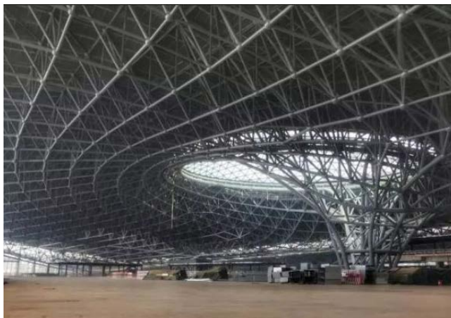
Figure 5. Construction site before ceiling installation 图 5. 吊顶安装前的施工现场
