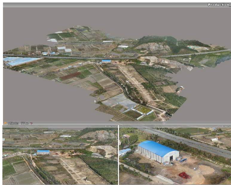
Figure 4. Overall and locally 3D real scene models of Xinsha Junction area 图 4. 新沙枢纽区整体及局部倾斜三维实景模型
