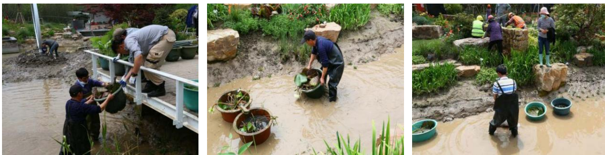
Figure 15. Water lily construction process: launching-positioning-planting
