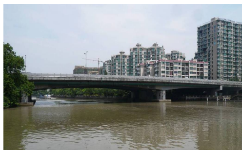
Figure 1. Yunhe Bridge 图1. 运河桥
