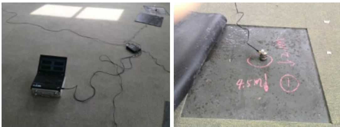
Figure 2. Measuring site 图 2. 测试现场情况
