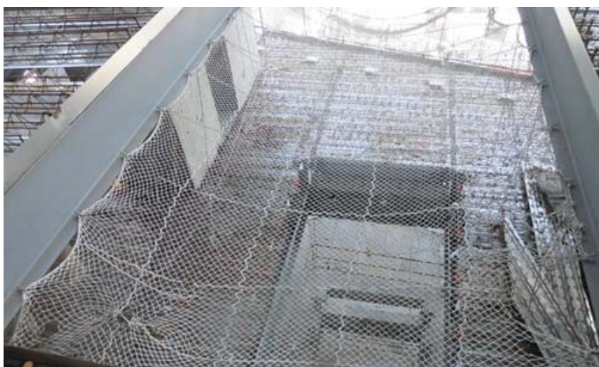
Figure 2. Level of safety net figure limb laid instance 图 2. 水平安全网临边铺设实例图
