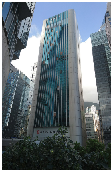
Figure 1. Curtain wall destroyed under strong wind
