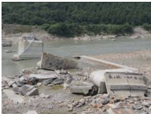
Figure 1. The collapse of the Jiangyou Panjiang Bridge in Mianyang City, China
