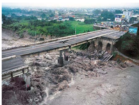
Figure 4. The ruined photo of the Houfeng Bridge in Taichung County, Taiwan 图 4. 台湾地区台中县后丰大桥冲毁照
