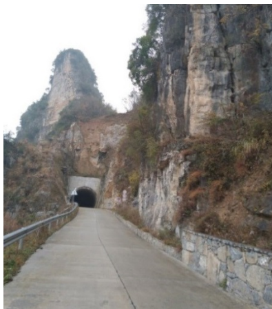
Figure 1. The situation of road tunnel exit 图 1. 公路隧道出口情况
