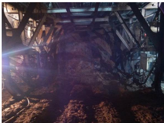
Figure 14. The picture of surrounding rock masses in Xiuwen Tunnel
