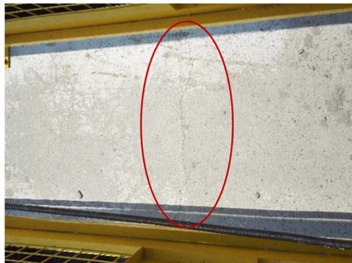
Figure 4. Cracks in concrete strut
