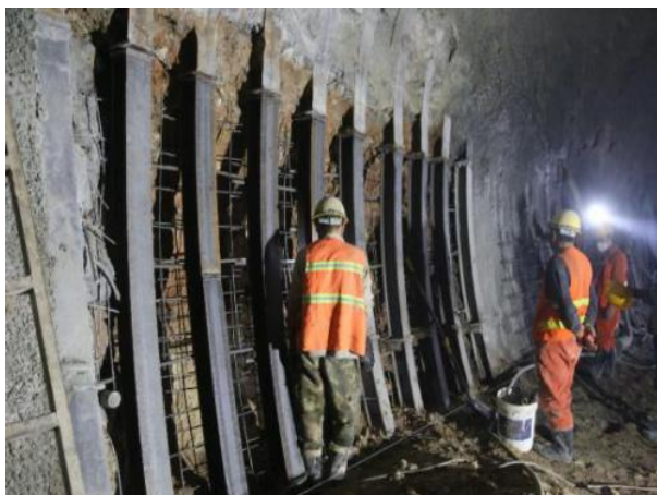
Figure 7. The on-site treatment—the side arch changing 图 7. 现场处理情况——换侧拱
