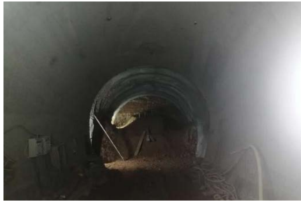
Figure 12. Secondary concrete in buffer layer section 2 图 12. 缓冲层段二衬混凝土 2
