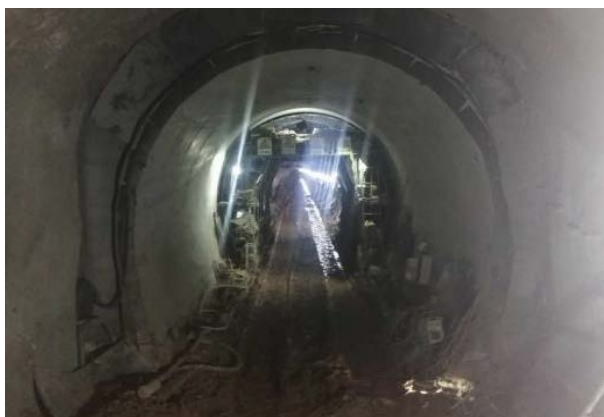
Figure 11. Secondary concrete in buffer layer section 1 图 11. 缓冲层段二衬混凝土 1
