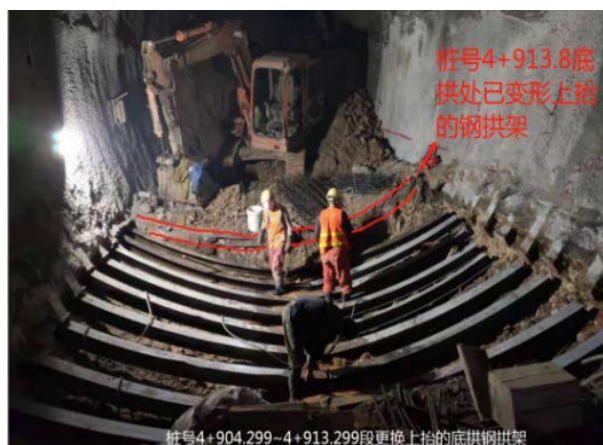
Figure 8. The on-site treatment—the inverted arch changing 图 8. 现场处理情况——换底拱
