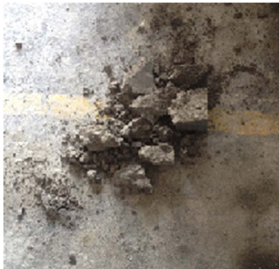
Figure 4. Test 1-5 96 hour state of concrete specimen
