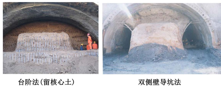
Figure 6. Bench excavation and side adit excavation—to leave the rock behind workface
