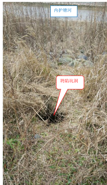
Figure 2. Current collapse pit points 图 2. 现状塌陷坑洞点
