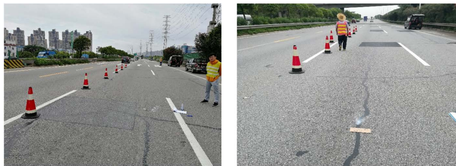
Figure 2. Difference of disease degree in different lanes 图 2. 不同车道病害程度差异
