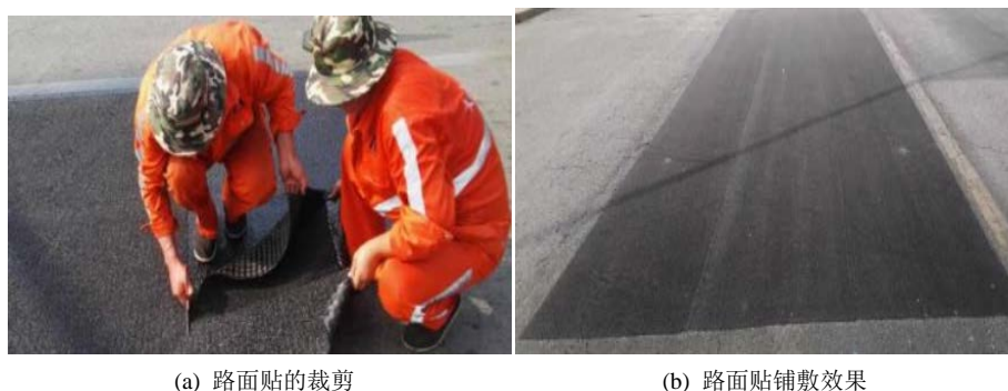
Figure 4. Application of pavement stickers 图 4. 路面贴的应用示例
