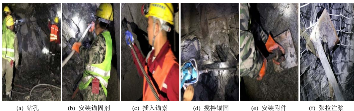
Figure 10. Birdcage anchor construction process 图 10. 鸟笼锚索施工工艺图
