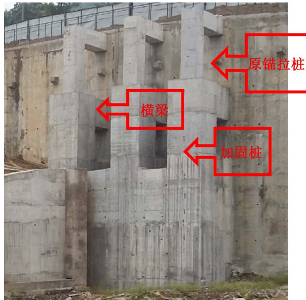
Figure 9. Slope deformation reinforcement structure real scene 图 9. 边坡变形加固结构实景
