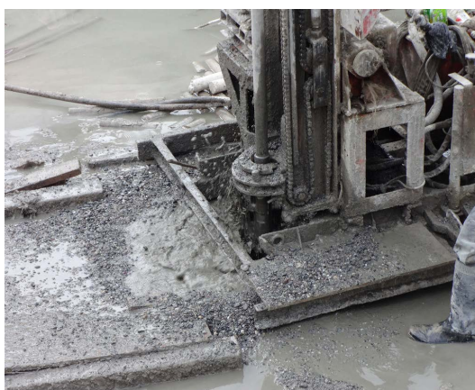
Figure 2. Construction pictures of high pressure washing hole
