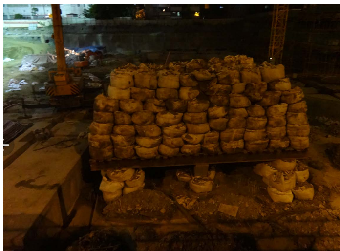
Figure 7. Disposal of dead load test site heaps
