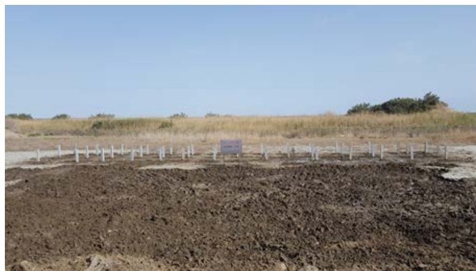
Figure 1. The completed test pile was buried 图 1. 埋设完成的试验桩
