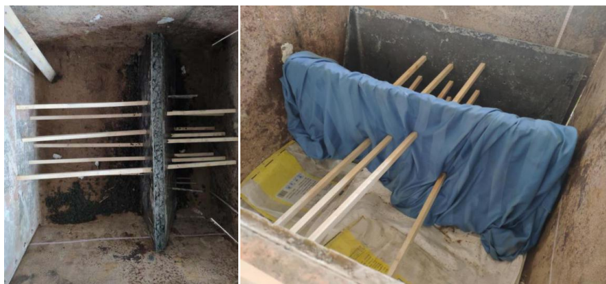
Figure 3. Pouring and maintenance of retaining wall 图 3. 挡墙的浇筑与养护
